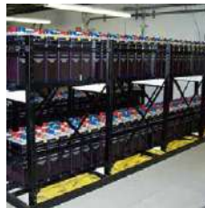
Server power supply
